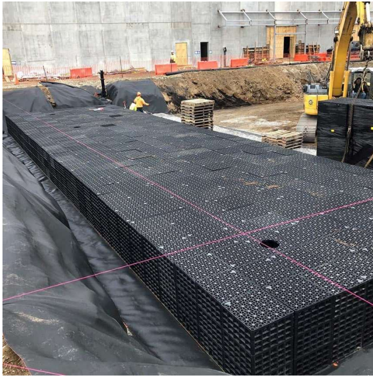
Figure 4: R-Tank being installed at a site for stormwater storage.
