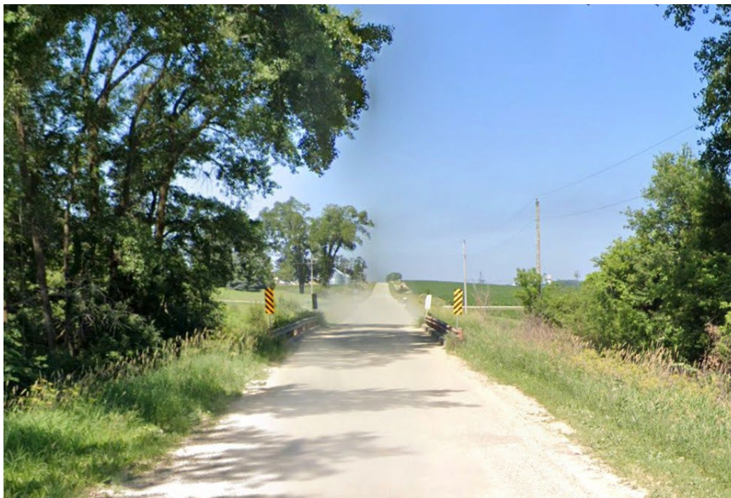
Figure 6T: 190th St Shared Use Bridge Westbound
