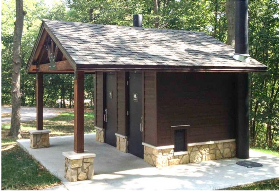
Figure 6E: Restroom Image
