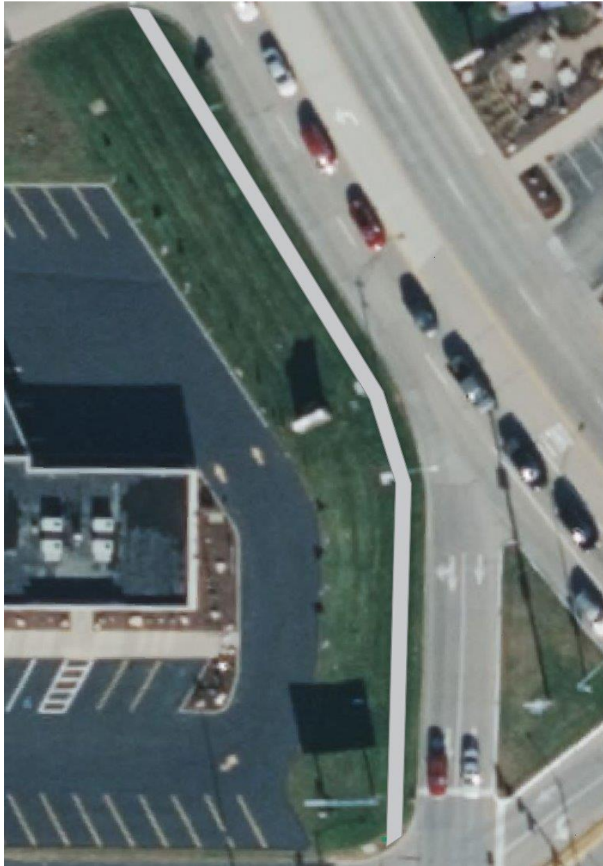
Figure 32. New Sidewalk Between Stoneman Rd and Wacker Dr
