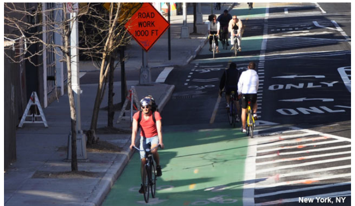
Figure 10. A cycletrak with clear markings (Source: National Association of City Transportation Officials)
