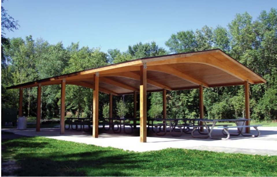
Figure 2: Image of a rectangular, open-air shaded structure from Poligon.
