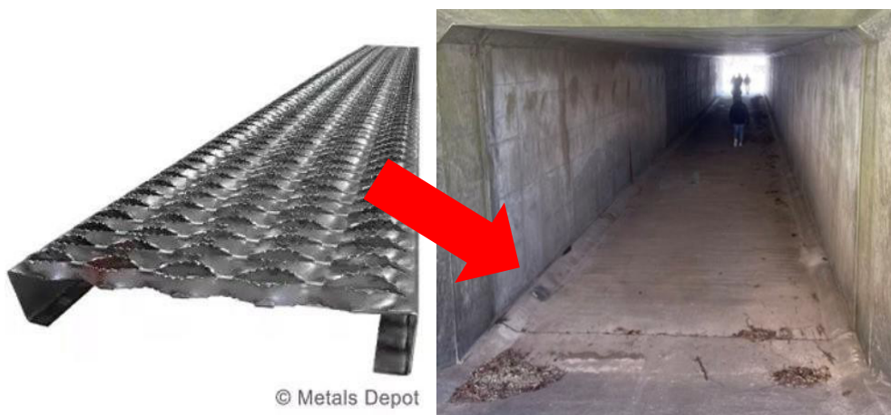
Figure 4: Existing culvert and proposed ground elevation technique.
