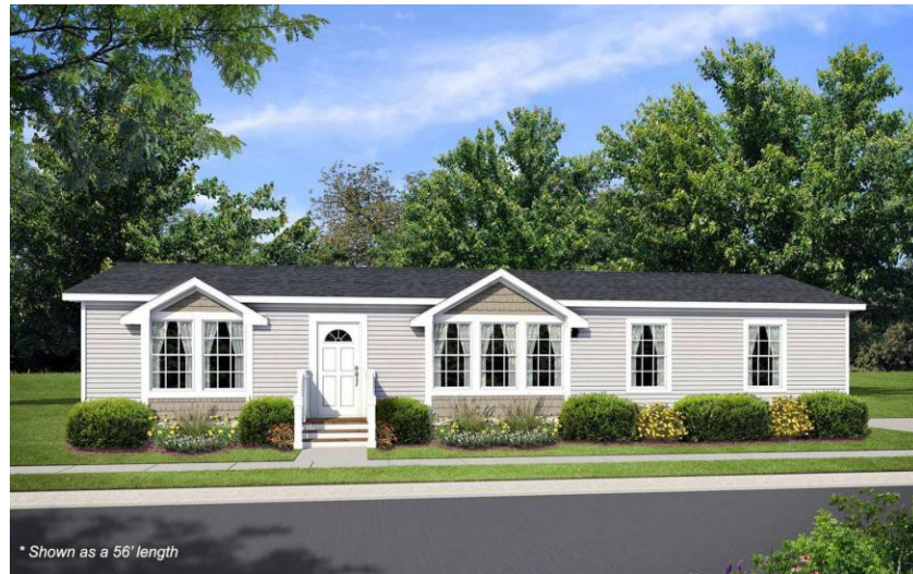
Figure 6.1: Example of a pre-manufactured home.
