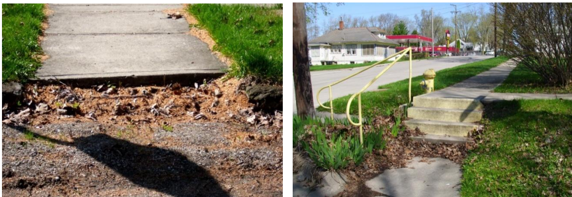
Sidewalk hazards like the abrupt ending (left) and stairs (right) make existing Wellman sidewalks difficult for the elderly and persons with disabilities. Photos: Jake Rosenberg & Sheila Knoploh-Odole
