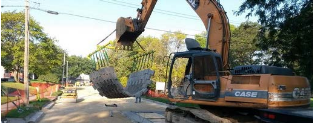
Figure 5-4. PaveDrain Installation.
