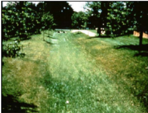
Grassed Swale Source: I ID Center
