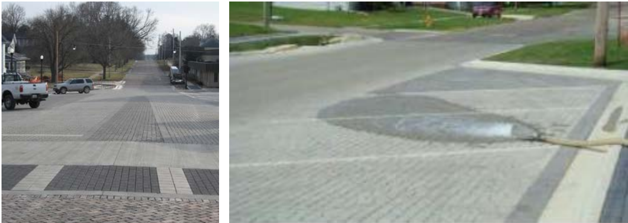
Figure 3-6. An example of brick pavers in West Union, Iowa (City of West Union, 2011)
