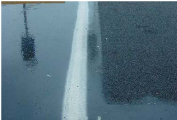
Figure 3-5. Comparison of traditional asphalt (left) and porous asphalt (right) when wet – (Hafner, Bassuk, Grabosky, & Trowbridge, 2007)
