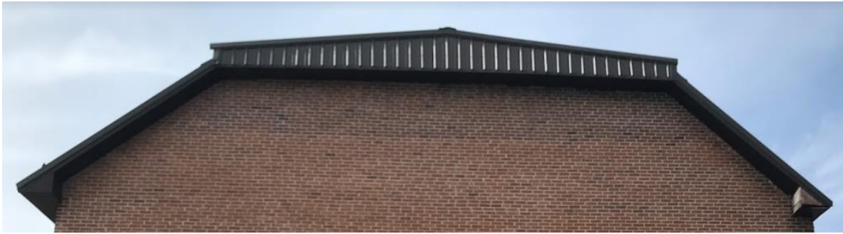
Figure 5. Current steel roof.
