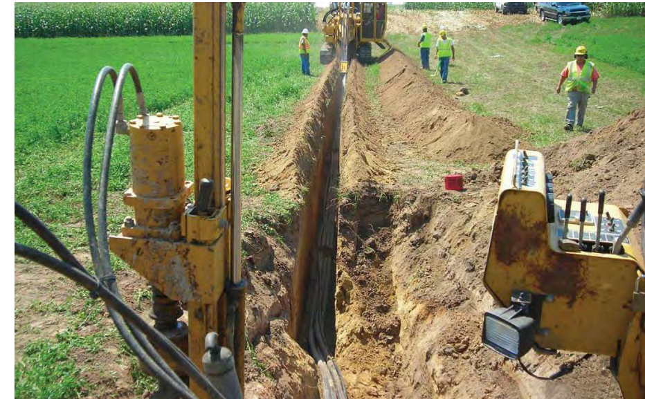
Burying the electric cables. Source: (WE Energies 2012)
