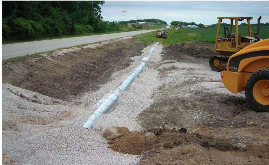
Laying out the culverts alongside the access road. Source: (WE Energies 2012)
