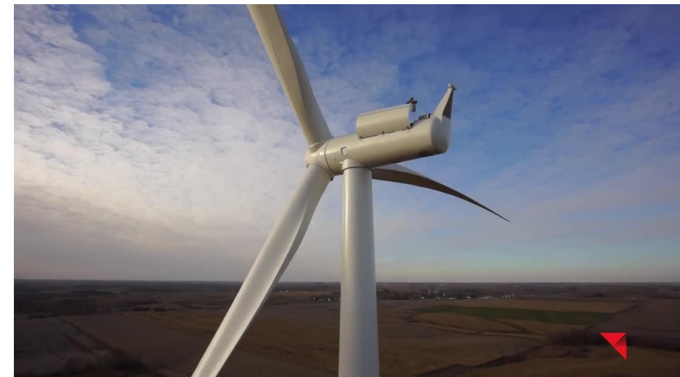
A newly constructed wind turbine. Source: MidAmerican Energy
