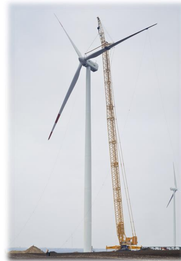
A crawler crane hoisting a wind turbine blade. Source: Liebherr
