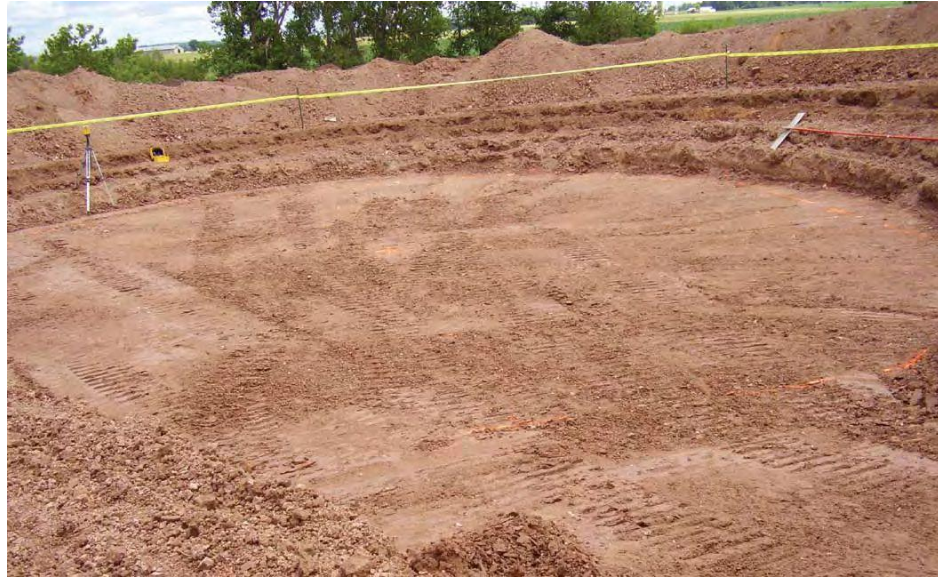
A prepared site for the wind turbine foundation. Source: (WE Energies 2012)
