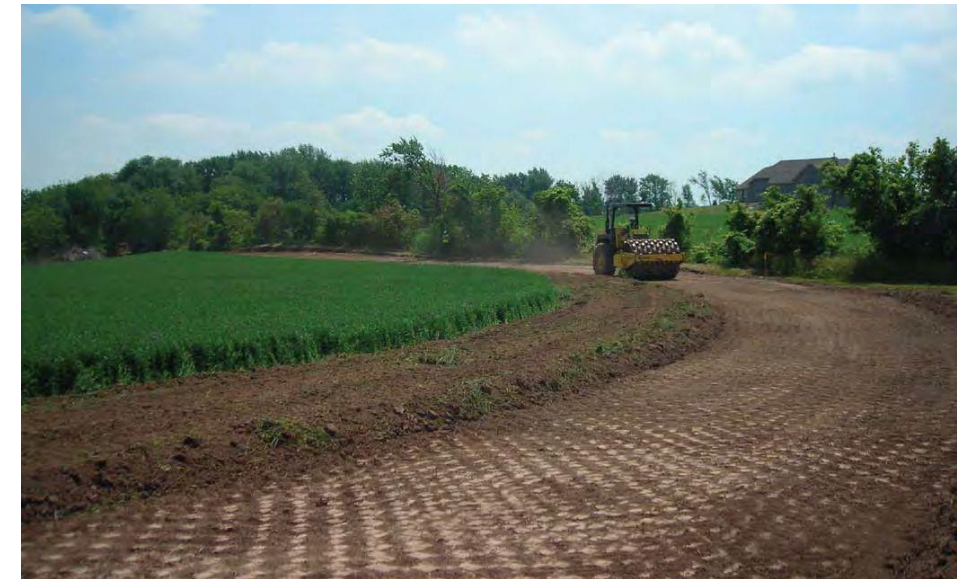
Laying out the geotextile matting. Source: (WE Energies 2012)
