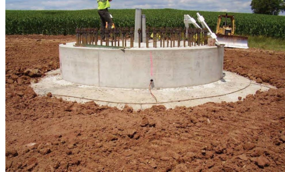
Covering over the completed wind turbine foundation. Source: (WE Energies 2012)
