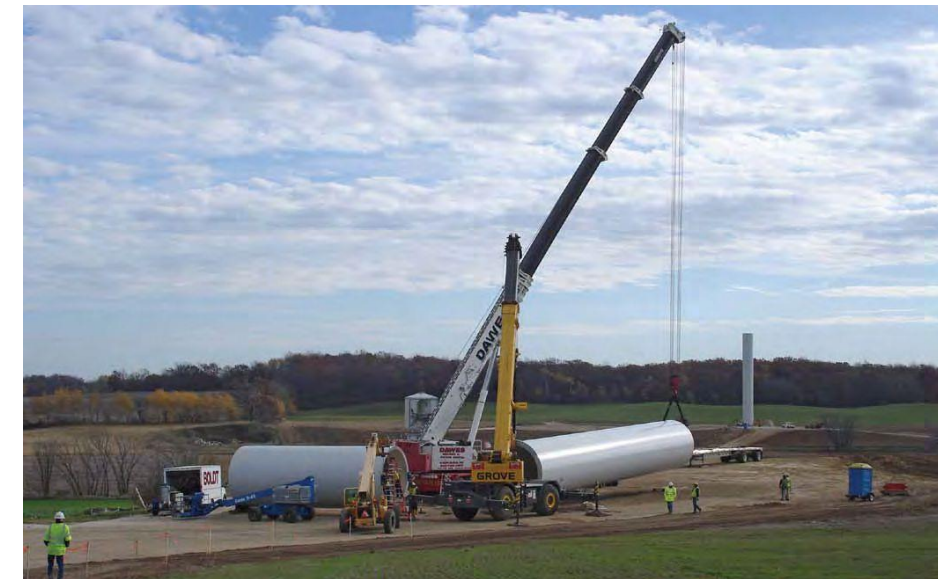
Erecting the other wind turbine tower sections. Source: (WE Energies 2012)
