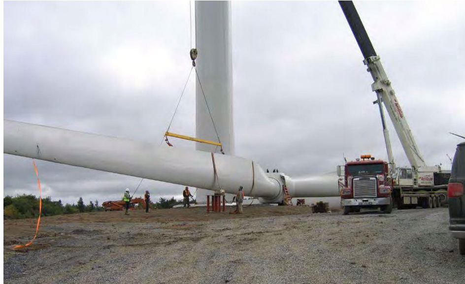
Installing the wind turbine blades onto the hub. Source: (WE Energies 2012)
