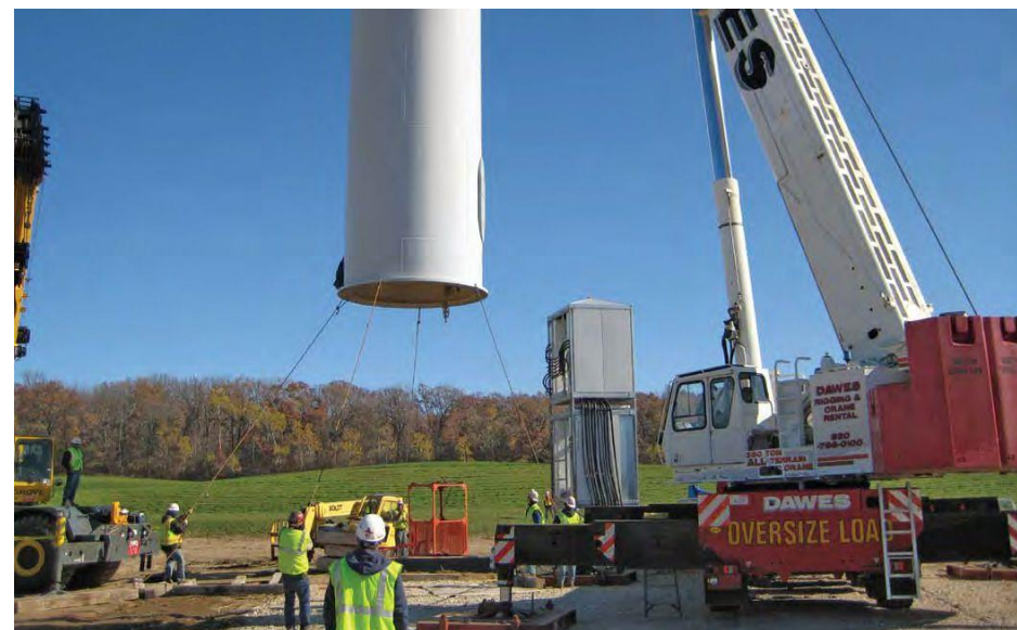
Erecting the base wind turbine tower section. Source: (WE Energies 2012)
