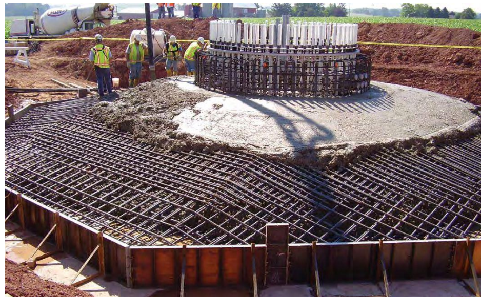
The concrete wind turbine foundation being constructed. Source: (WE Energies 2012)
