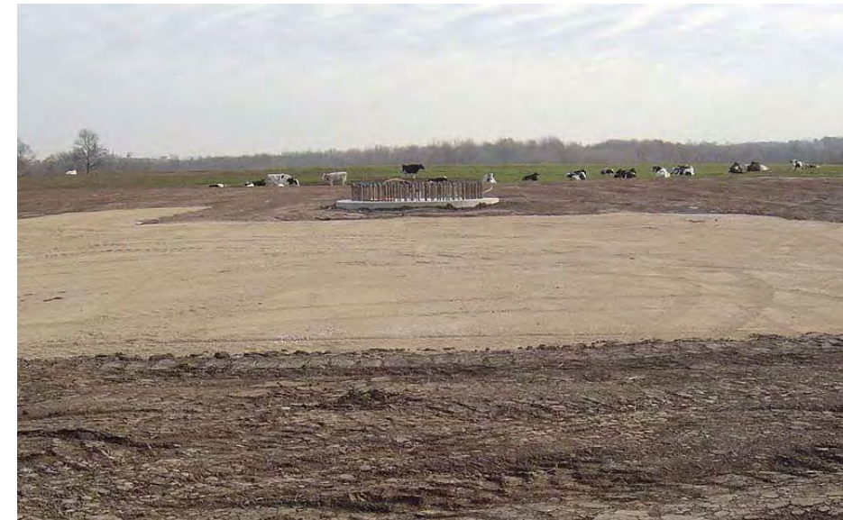
A crane pad near a wind turbine foundation. Source: (WE Energies 2012)
