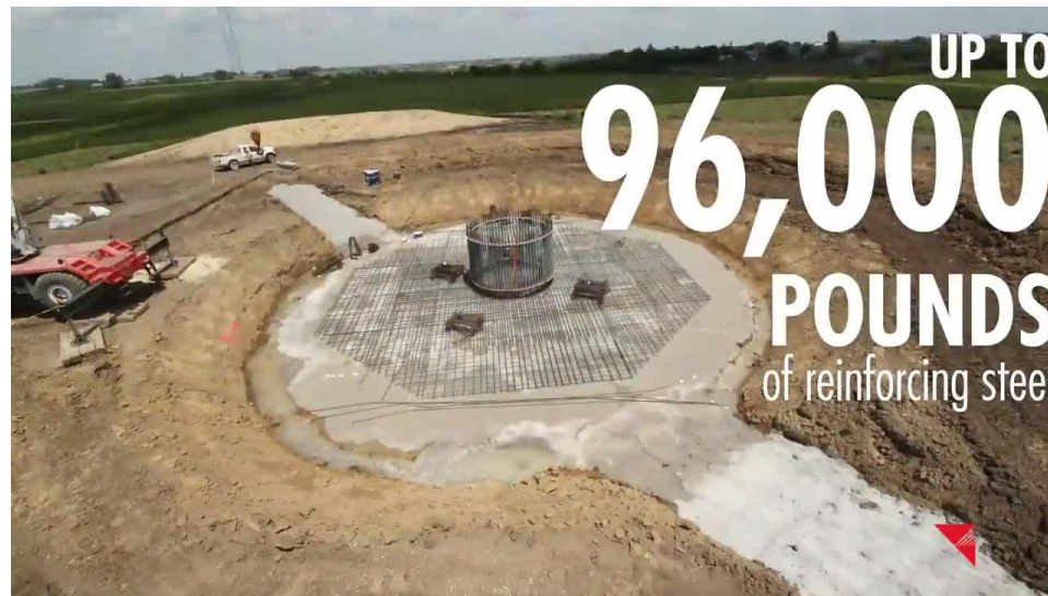
The rebar for the wind turbine foundation. Source: MidAmerican Energy
