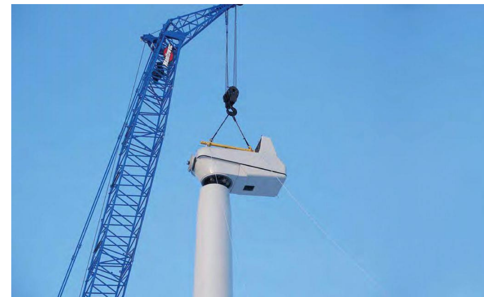
Lifting the nacelle onto the wind turbine tower. Source: (WE Energies 2012)
