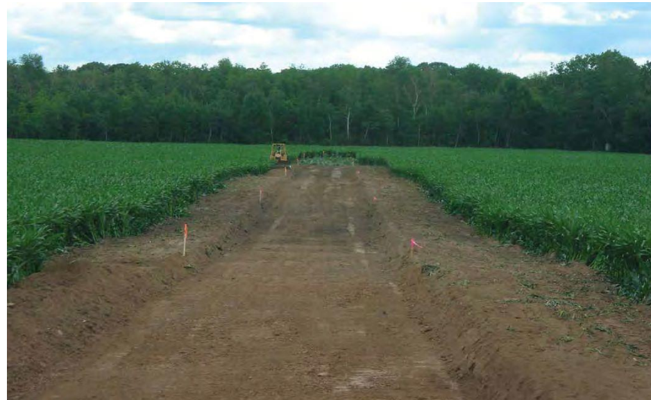
Initial site clearance and temporary road access. Source: (WE Energies 2012)
