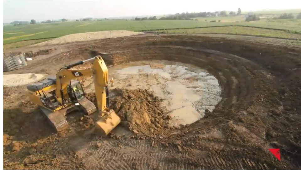
Excavation for the wind turbine foundation. Source: MidAmerican Energy
