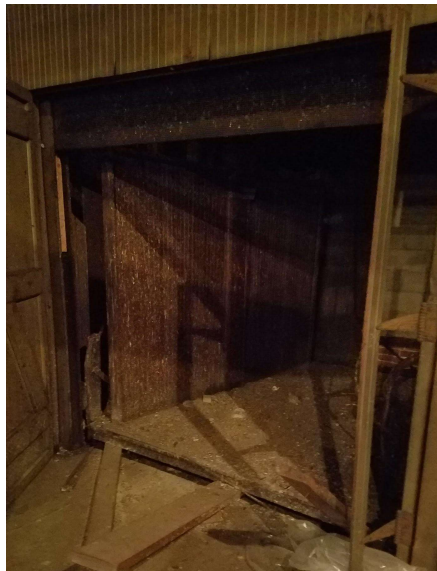
Figure 4. Current Elevator Shaft Found in the Brown Building
