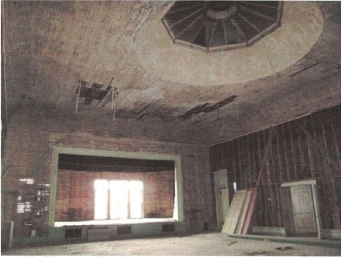
Figure C-5. Existing Ballroom Condition on the Third Floor of the Jacobsen Building
