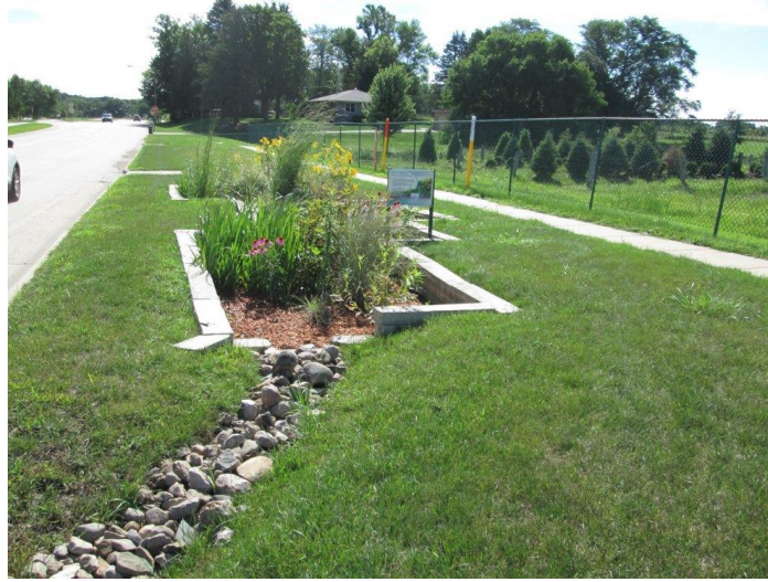
Figure 1.1: Vision for Bioretention Cell
