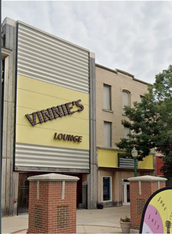
Face of Buildings
