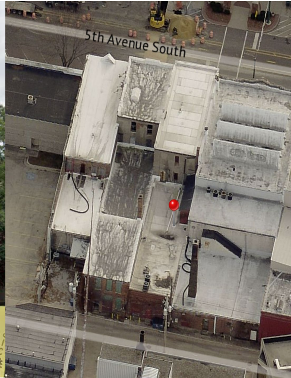
Rear View of Buildings
