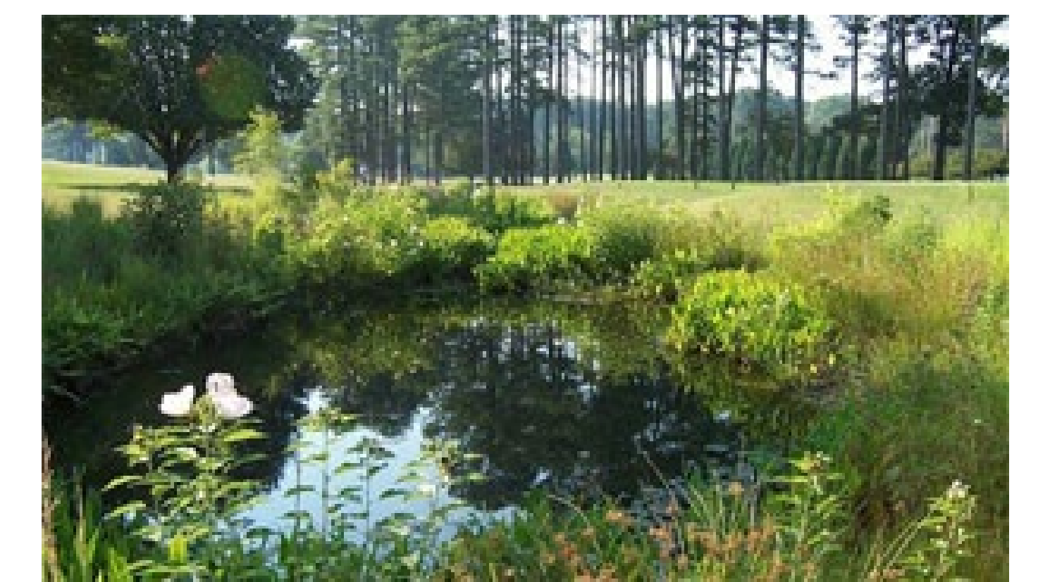
Figure 4.2 - Example of a constructed wetland.
