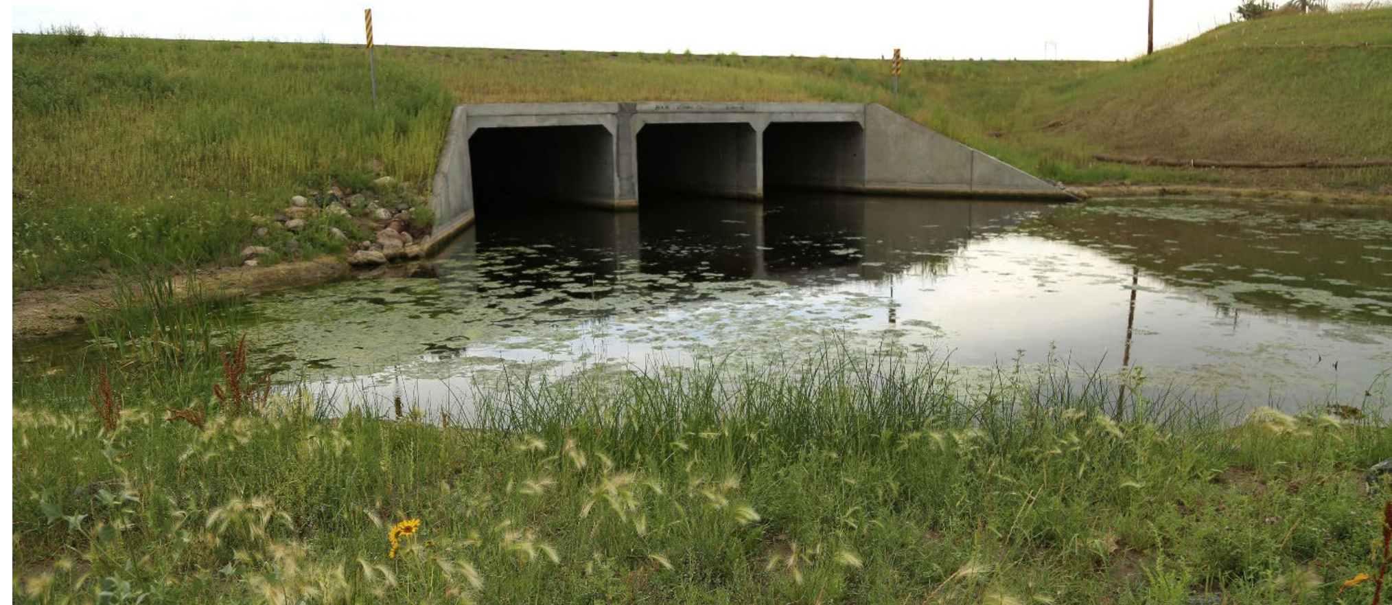
Figure 2. Box culvert example
