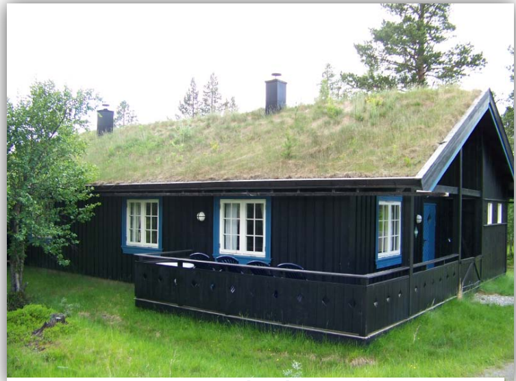
Figure 16: Residential Green Roof
