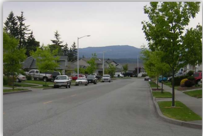
Figure 10: Excessively Wide Residential Street
