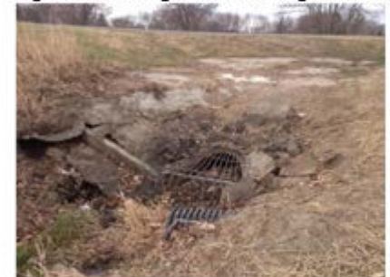
Figure 3: Existing culvert at the outlet
