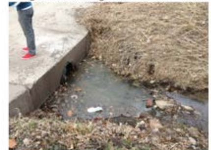
Figure 4: Existing culvert under west main street
