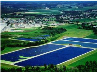
Figure 4: A wastewater treatment lagoon with submerged aerators
