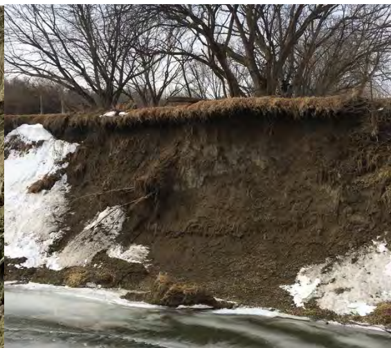
Figure 3b: Shear walls of erosion
