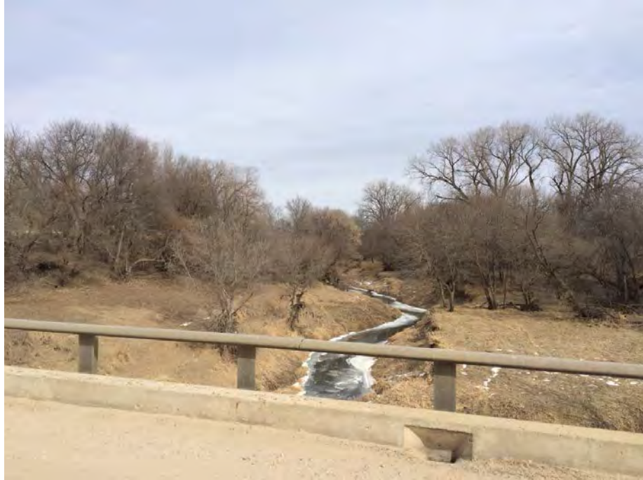
Figure 4: Site of S. Ridge Rd. dry detention basin
