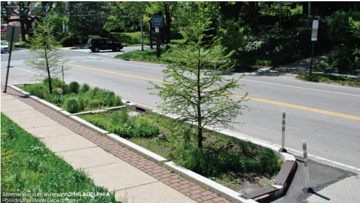
Figure C3. Example bump-out with curb cut in middle of bump-out allowing water to flow from street
