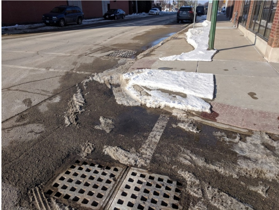
Figure 14. Typical location of storm water inlets are at corners of intersections. A traditional bump-out would impede these inlets.
