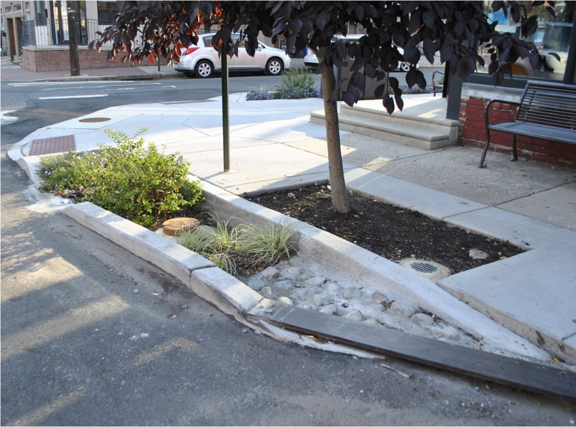
Figure C2. Example bump-out with curb cut to allow water to flow into the bump-out but still restricts vehicular and bicycle traffic.
