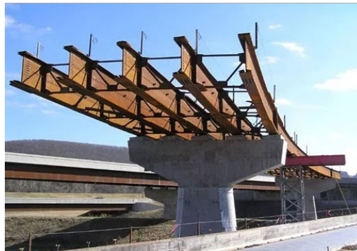
Figure 4.1.3: Steel Plate Girder Bridge Concept
