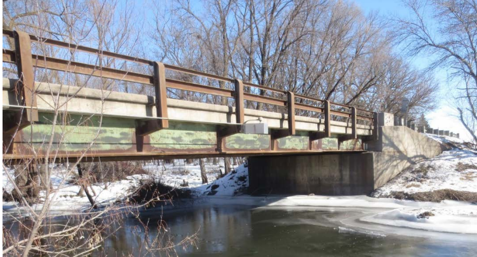
Figure 4.4.2: Existing Willow Creek Bridge.
