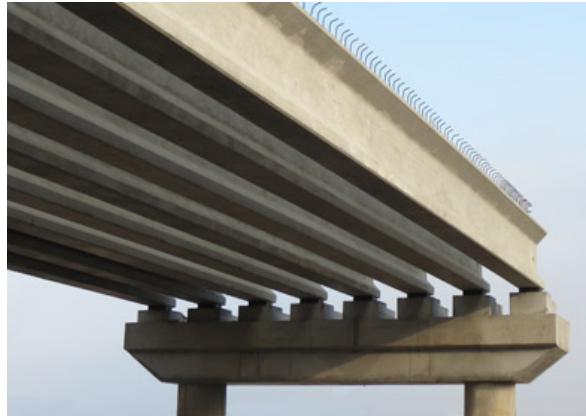
Figure 4.1.2: Pre-stressed Concrete Bridge Beams Concept
