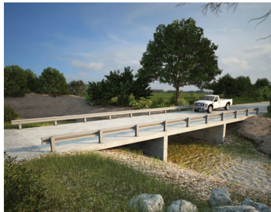
Figure 4.1.1: Pre-cast Concrete Slab Bridge Concept
