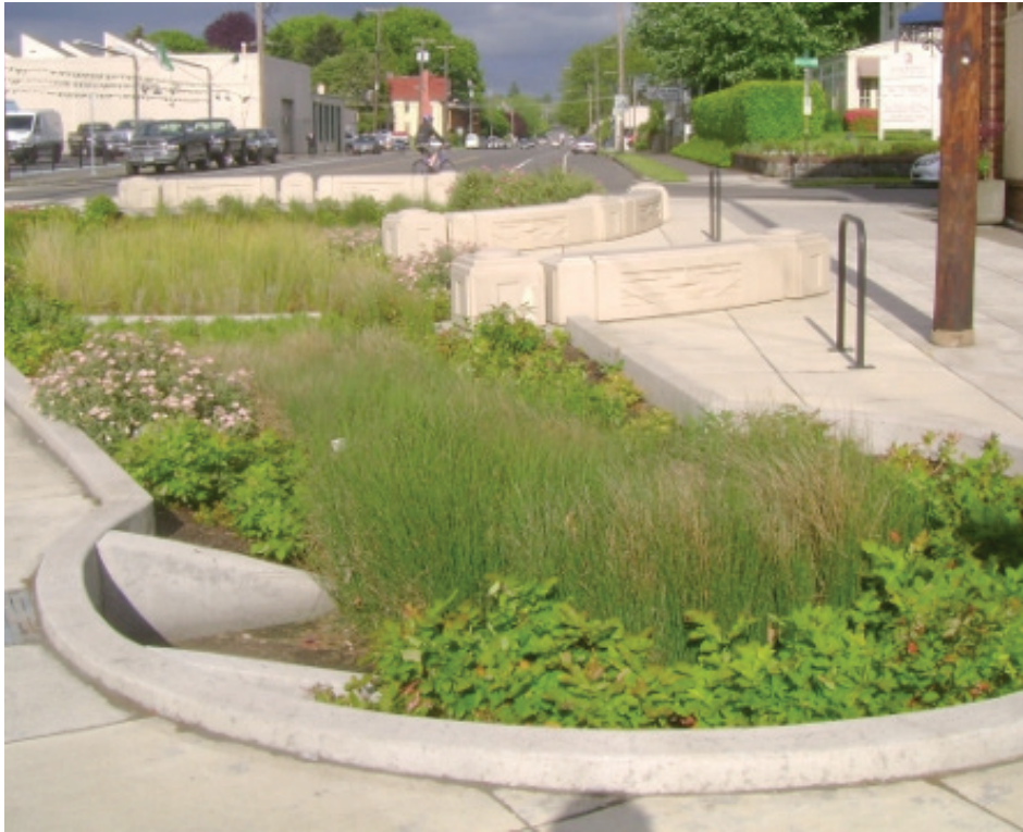
Figure 49. Urban rain garden. Source: South Side Green Infrastructure Charrette.
