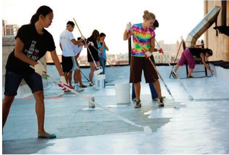
Figure 4. Painting white on the roof of a commercial building. Source: nationswell.com
