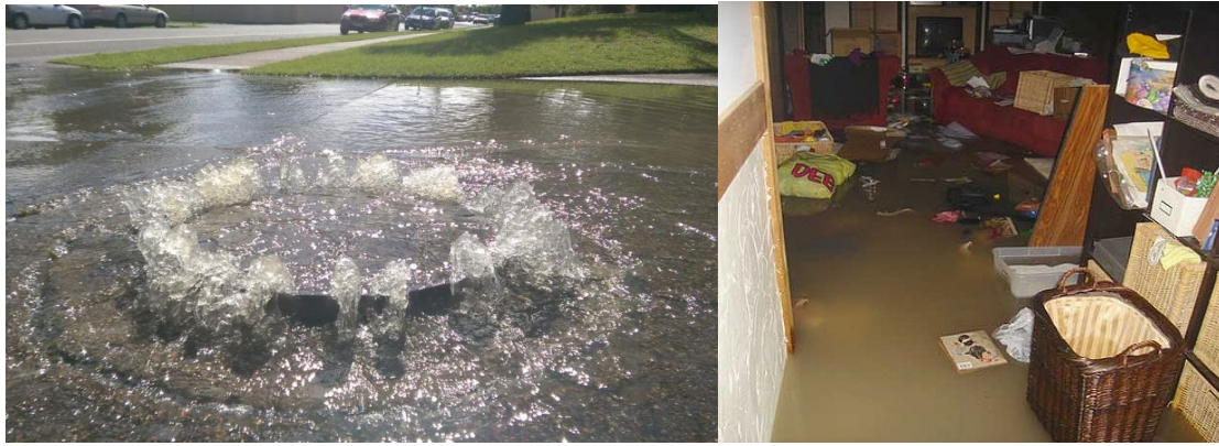
Figure 1: Overflowing manhole and basement backup
