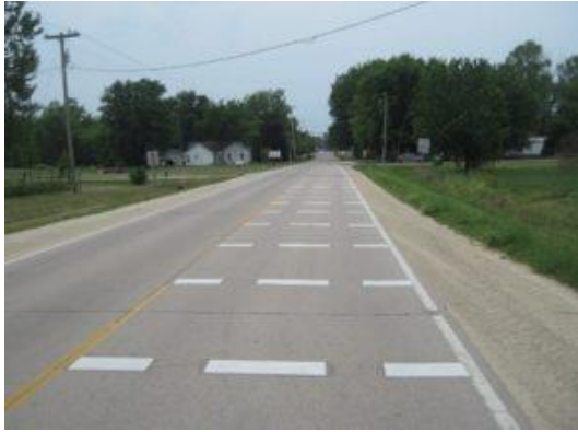
Figure 20 Transverse roadway marking example
