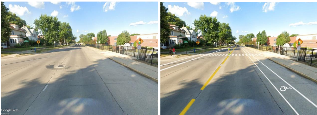
Figure 17: 5th Street Recommendation 2 Option 1, two-way road diet and redesign
