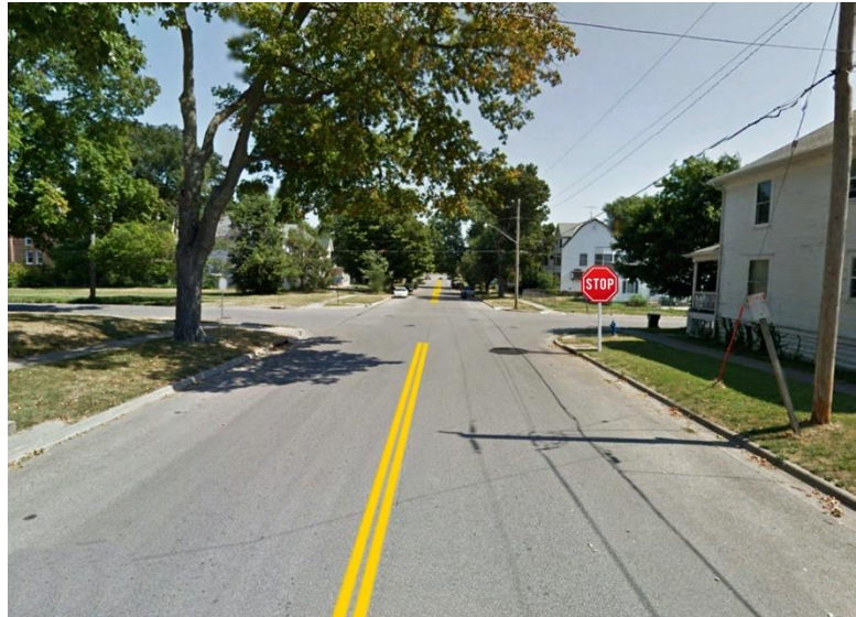
Figure 15: Future 3rd Street with painted yellow line and stop sign.
