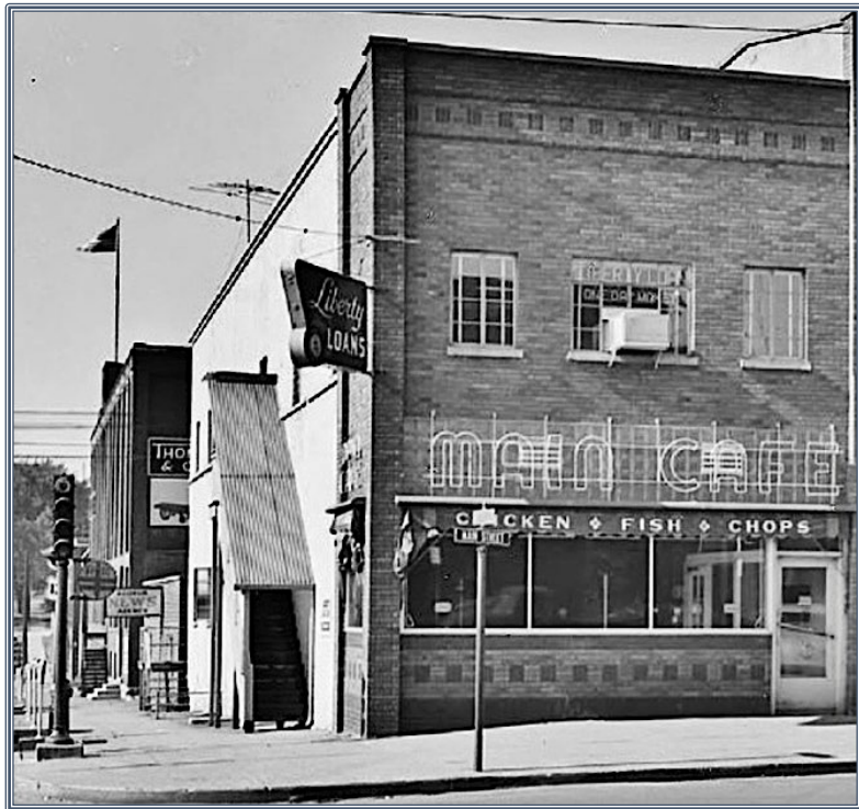
The Main Street Café was demolished after the 2 nd floor collapsed into the 1 st and the building became unsafe to passersby (Keokuk Historians, 2020).
