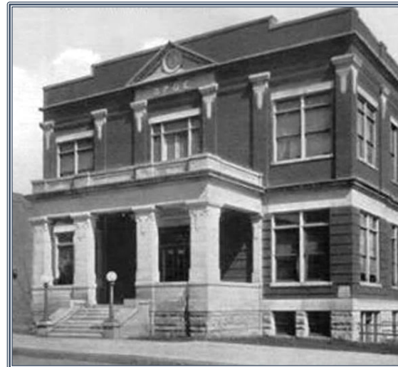
The former Elks Lodge at 601 Blondeau Street circa 1930. Source: Keokuk Historians
