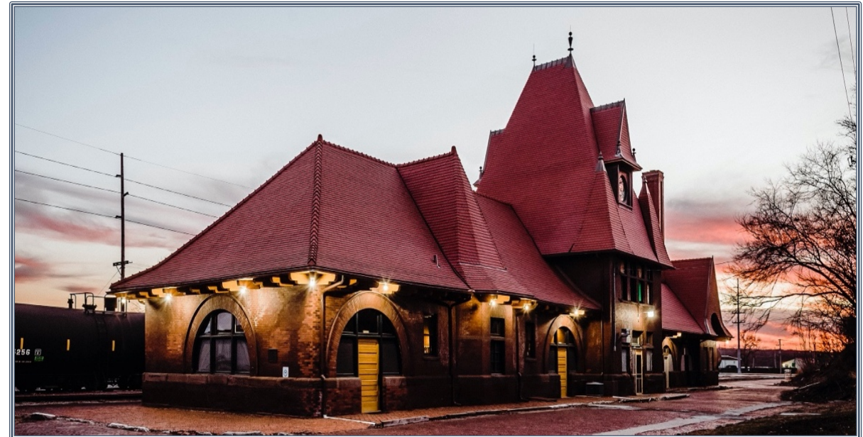
No longer a depot proper, the Keokuk Union Depot is hidden to the south by three rows of railcar storage and to the north by a bluff. Photo by: Allen Consulting Group
