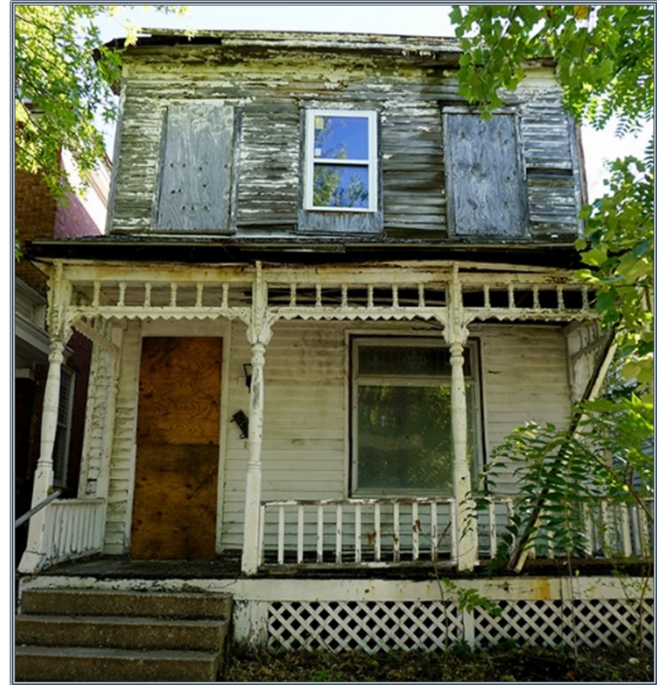
Dilapidated and possibly abandoned housing on 10 th Street. Source: Authors.
