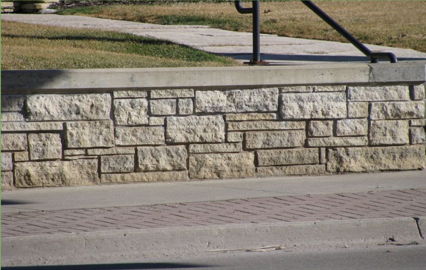
Fig. 9. Poured in place concrete retaining wall with limestone veneer located in Iowa City, IA.
