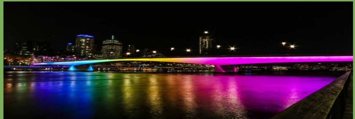
Fig. 5. Bridge lighting example of Victoria Bridge in Brisbane, Australia.
