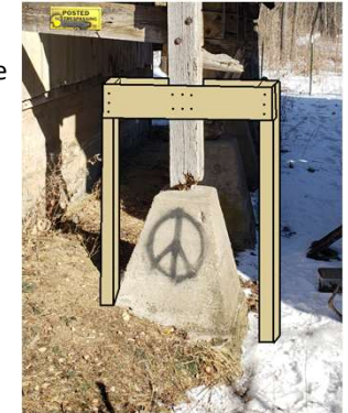
Figure 8 – Temporary Lumber Supports for Rock Crusher Columns
