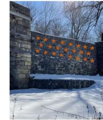
Figure 5 – Soil Nailing Layout
