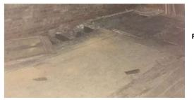
Figure 7. Floors will be removed and replaced due to deterioration.
