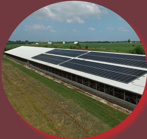
Solar Panels on a Turkey CAFO. Source: Iowa Farm Bureau, 2017.
